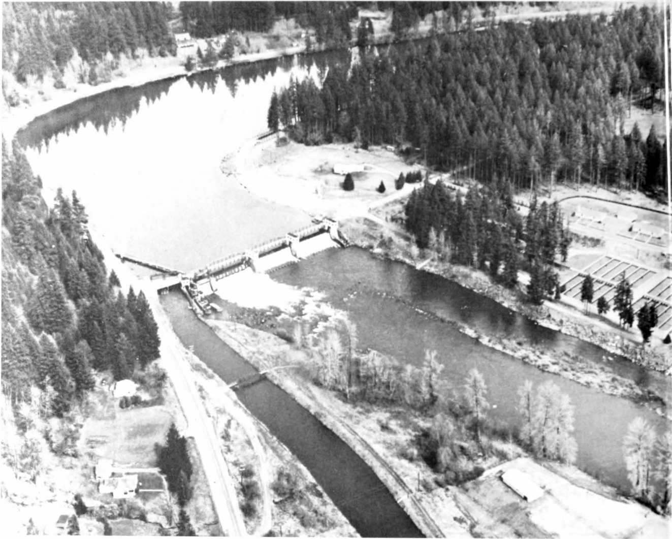
Figure 6.—Upstream view of the McKenzie River, showing the Leaburg diversion dam and canal.
